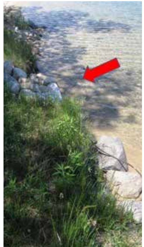
Drainage culvert emptying into Crystal Lake
