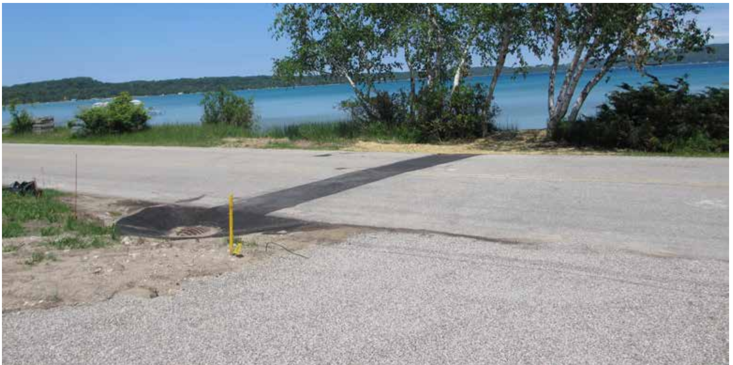
Newly installed drainage culvert under South Shore Road
