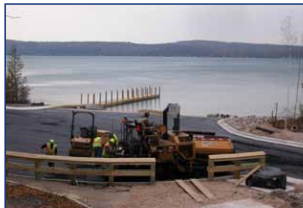
Paving crews finish work on the boat launch site in November.
