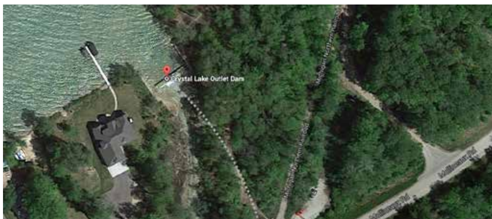
Location of Crystal Lake Outlet dam from air (Google Earth)
