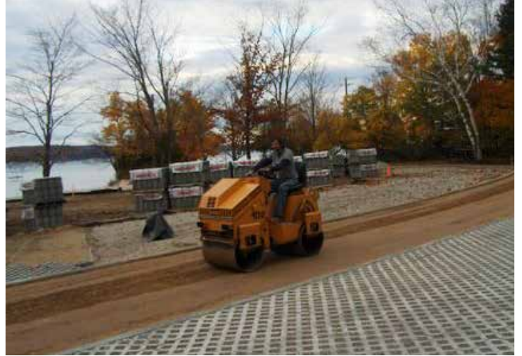
Constructing park road and parking area, November 2016 (photo: E. Hill)
