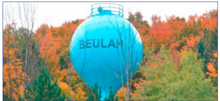
New water tower, fall 2018
