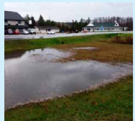
Catch basin west of US-31 near BP station in Beulah
