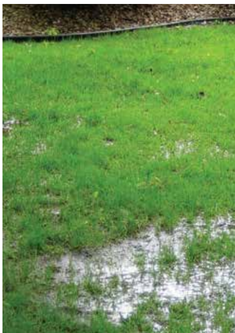
Lawn with failing septic system
