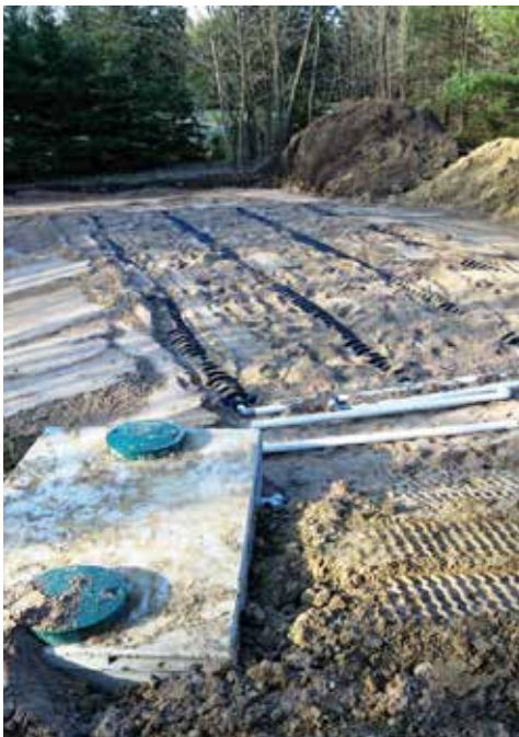
Drain field under construction
