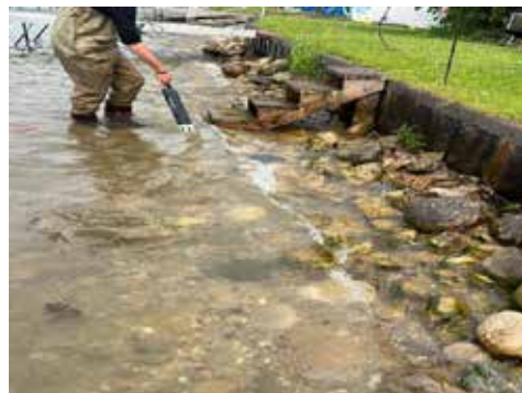
Figure 3. Hardened shoreline: sea wall and riprap
