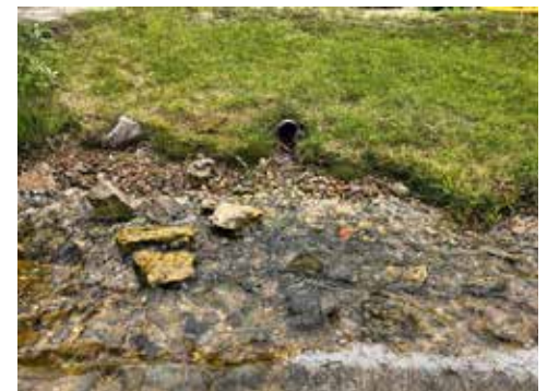
Figure 4. Green lawn to shoreline (no vegetative greenbelt), drainage pipe
