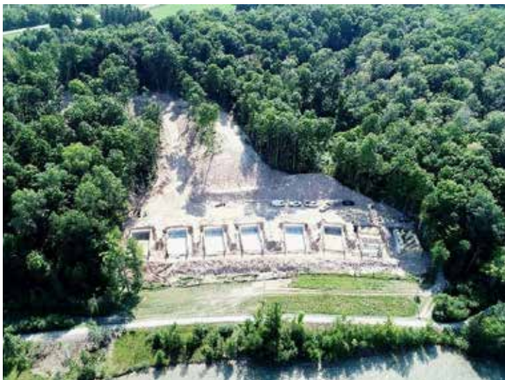
Sunkissed Hills site after clearing, foundations laid (August 2022)
