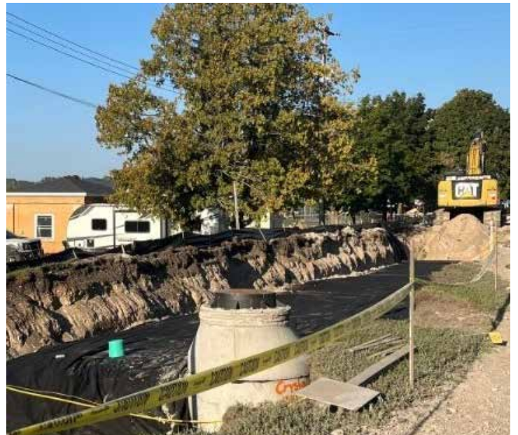
Stormwater remediation construction along Betsie Valley Trail, fall 2025
