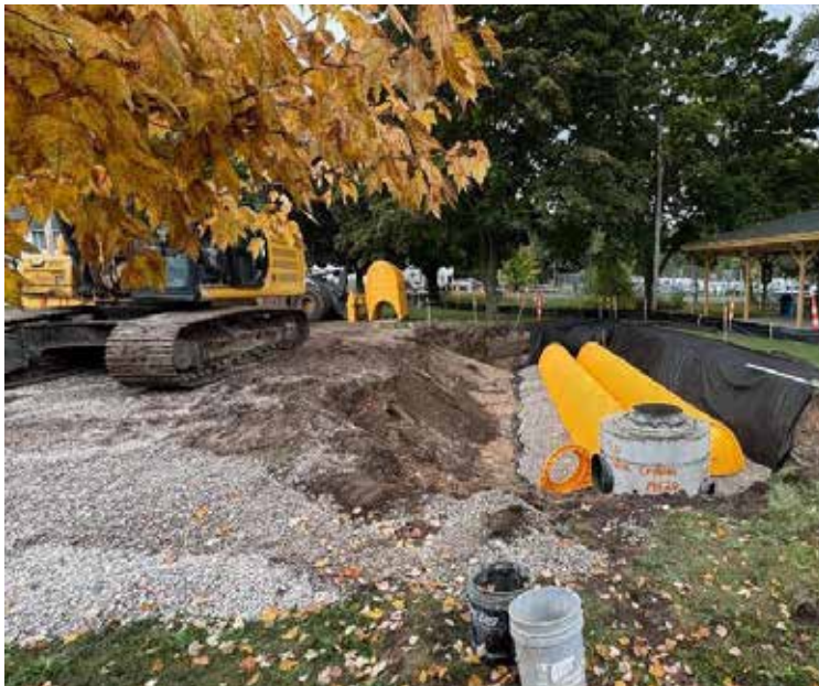
Stormwater remediation construction in Village Park, fall 2025
