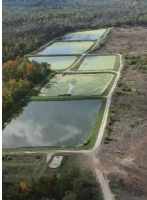
Lagoons serving as treatment for Beulah's wastewater
