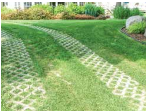
Permeable driveway on South Shore
