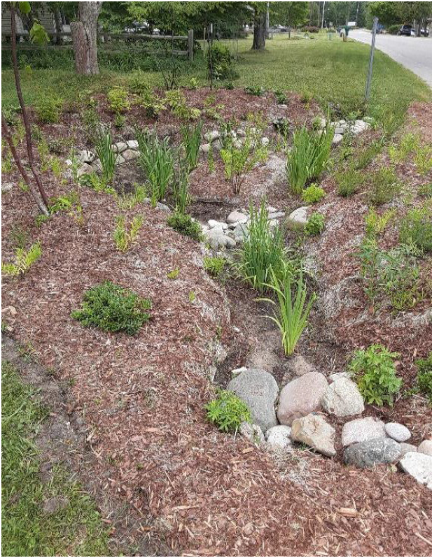
This beautiful rain garden keeps dirty water runoff from flowing through a culvert into Crystal Lake.
